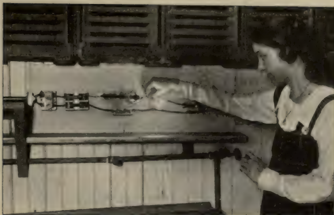
FIG. 131. Feeling one live wire does not give her a shock, but what would happen if she touched the gas pipe with her other hand?
